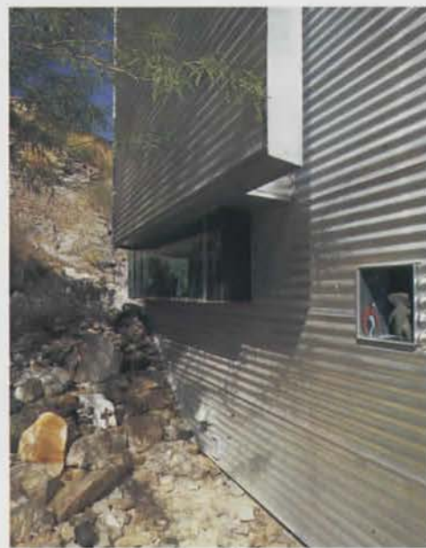
ABOVE The angular laundry-room window is as much a part of the composition as every other opening in this iconoclastic home. A hanging corrugated panel detached a few inches from the wall allows light into the second-level master bath.
