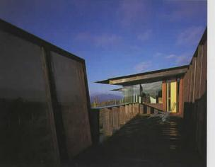
The main floor plan (below) and east elevation (above) show the organization of the internal space around a linear spine' made of concrete-block walls learning at varying degrees from the vertical and horizontal (opposite right, above and below). A steel-framed roof is cantilevered off the 'spine' and juts out over the main living spaces towards the front of the brace (see elevation).
