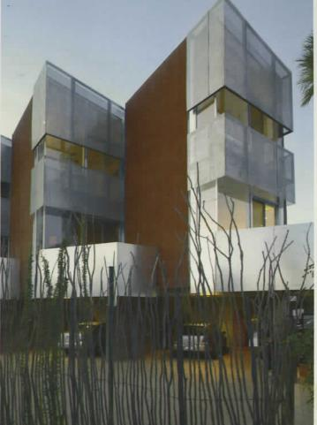
surrounding landscape. Corrugated steel is used in addition to sandblasted concrete masonry and zinc cladding, some of which was allowed to rust to create a colour palette appropriate to the desert setting.
