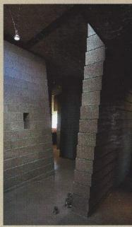
"Canyons" that slope to the lower level (top) and create a circulation spine for the main floor (right) seem to be shaped by geologi cal forces. The concrete blocks in the canted interior walls are laid in courses parallel to the angled roof, not the floor. Rebar runs vertically through each concrete-block cell and across every third course. Glass orbs are by artist Mayme Katz.
